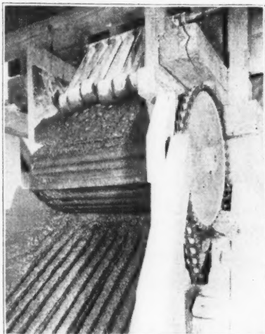
Feeder Below Car Dump. The Inclined Bar Grizzly Takes Boulders to Crusher.
